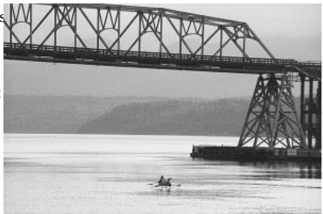
Hood Canal Bridge
